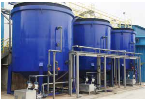
Advanced Dissolved Air Flotation (DAF) clarifier for chemical treatment
